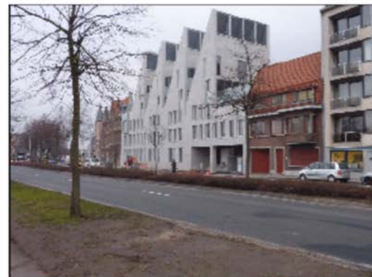
Apartment project realisation "Gulden Vlieslaan" (Source: City)
